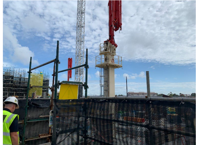
Photo 2: General Construction and Dust Shadecloth
